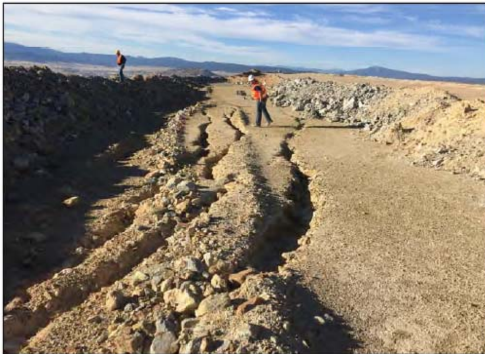
Photo 4. Cracking reported in the 2016 AIR report on the North-South Embankment.
