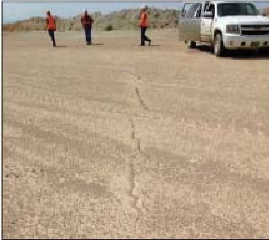
Photo 3. Cracking typical of a Riedel shear system.
