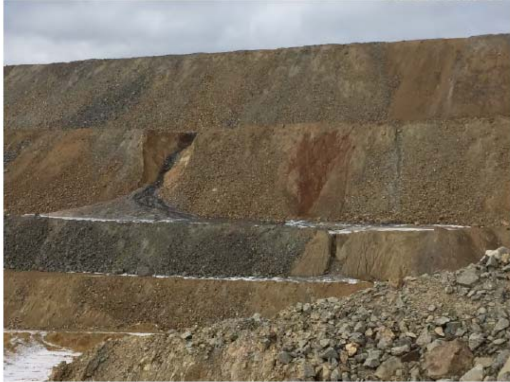
Photo 2. Seepage incident on North-South Embankment reported in 2016 KP EOR report.
